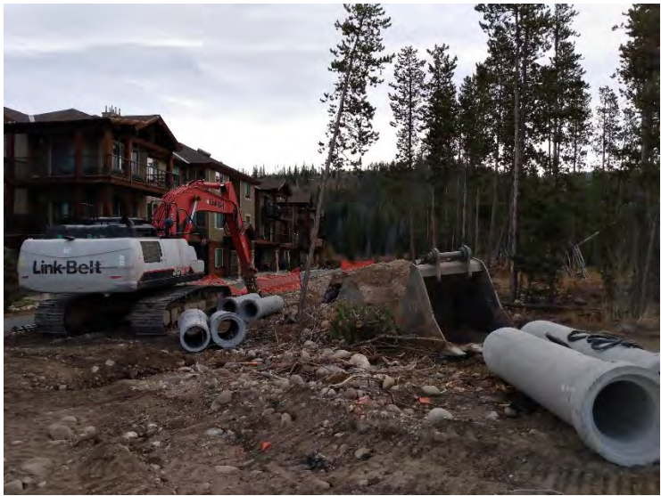
Storm Sewer West Boundary
