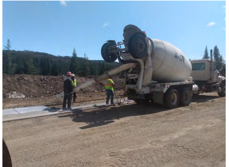
Placing Sidewalk
