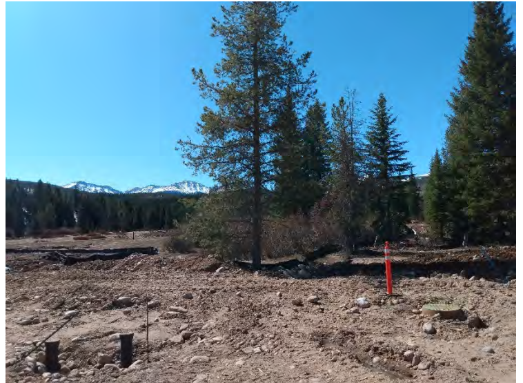
Southeast View from Roundabout
