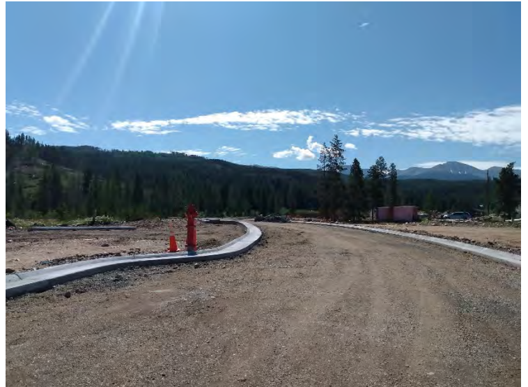
Curb and Gutter
