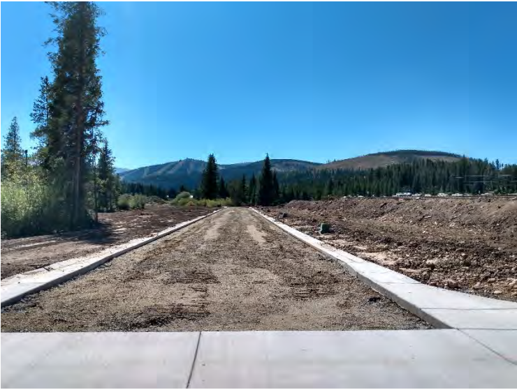
Curb and Gutter
