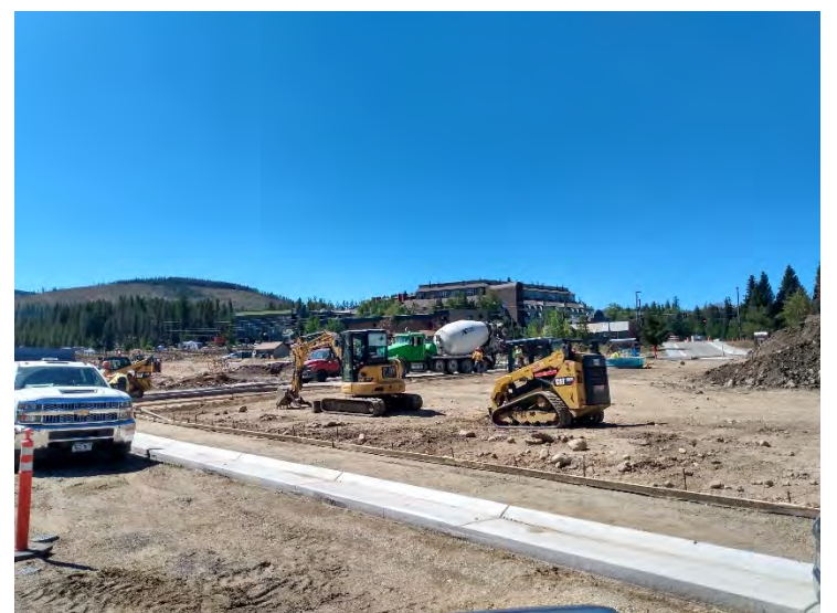
Curb and Gutter
